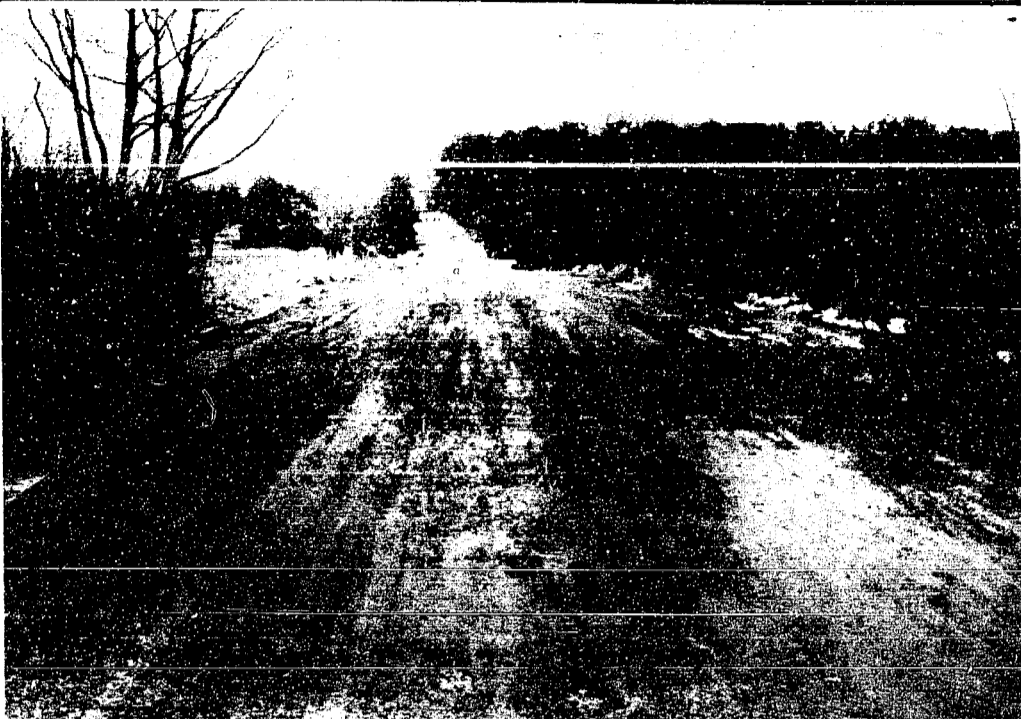
TRINKLE RD. was open to through traffic between Fletcher and Freer Rds. early this week after road commission workers put down the final layer of a light-weight, blast-furnace slag. While commis-
